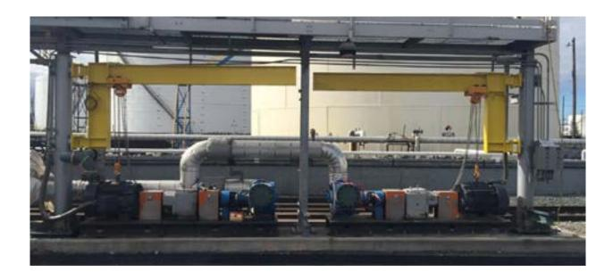
Tikal crane system in a pump station is a vital tool for handling the installation, maintenance, and repair of heavy equipment, particularly pumps. The type of crane system chosen depends on factors such as the layout of the pump station, available space, and specific lifting requirements. The crane system plays a crucial role in ensuring the reliability and efficiency of pump operations within the water treatment facility.
